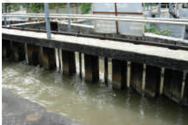
Fig. 18.4 Grit and sand removal tank
