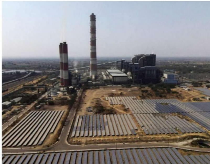
A drone view of solar panels and the NTPC (National Thermal Power Corporation) power plant in Solapur, Maharashtra. REUTERS
