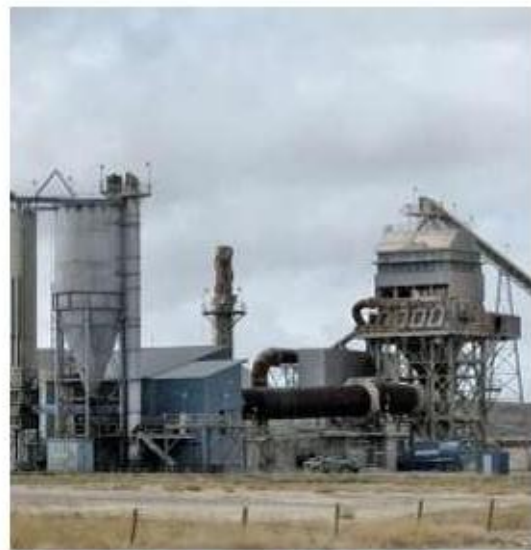
A rotary kiln is visible as the rust-coloured horizontal tube at the centre in this image of a cement plant in the U.S. GREG GOEBEL (CC BY-SA)
