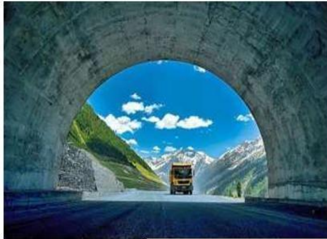
The Zojila Tunnel is likely to allow security officials to ferry goods to the high-altitude bases of Ladakh during peak winter. ANI
