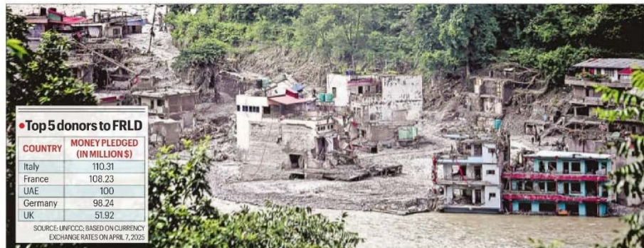
The devastated structure around Betrawati Rasuwa border in Nepal following the flash floods on August 31. FILE
